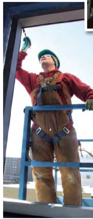
Sparks fly as Foothills Acoustics' Jeff Fichtner trims a steel stud for installation.
