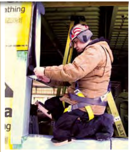
Bending metal is easy for Travis Mercredi MacDonald, an electrician with Ryfan Electric, as he prepares electrical conduit for installation.
