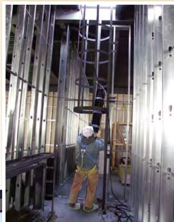
Gordon Snow with Unico Roofing Contractors guides a roll of vapour barrier to the roof of the Gallery Project construction site.
