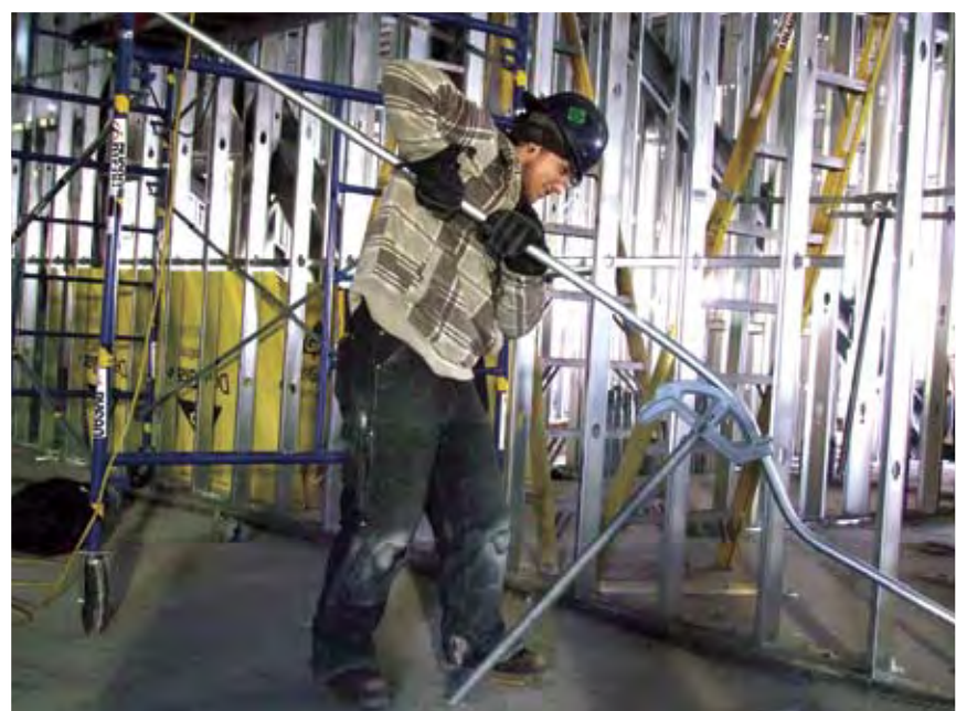
Bending metal is easy for Travis Mercredi MacDonald, an electrician with Ryfan Electric, as he prepares electrical conduit for installation.
